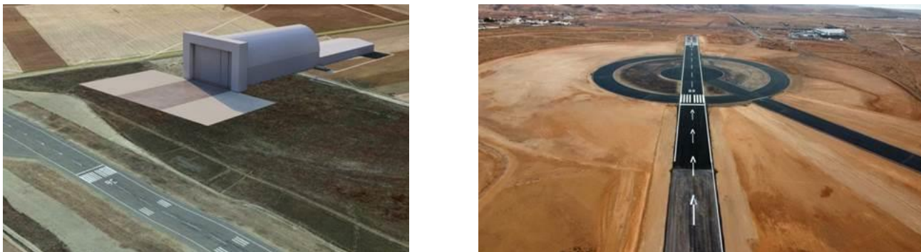
Figure 5: airship HAPS facilities at Teruel airport (left), Fuerteventura stratoport (right)
